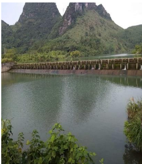
(c) 库区及大坝全貌
