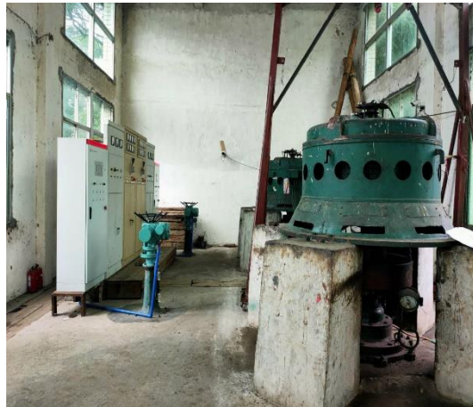
(b) 厂内发电机电层
